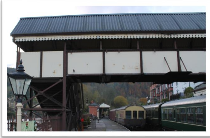
The top deck of Llangollen Station footbridge. In these photos the separate beams supporting the side panels and the roof are clearly visible.
