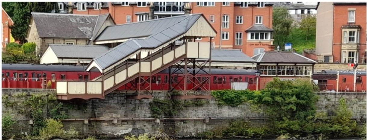
The station footbridge at Llangollen; note how the steps extend over the River Dee, supported by gantries and a landing platform, which themselves are supported on steel beams cantilevered out from the retaining wall.
