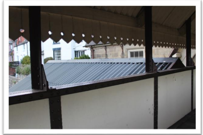
The top deck of Llangollen Station footbridge. In these photos the separate beams supporting the side panels and the roof are clearly visible.
